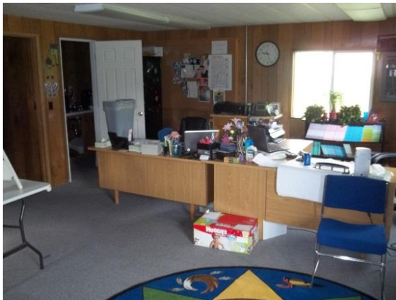
Culture Building (102T) – Classroom 5 Original floor covering has been hidden by wall-to-wall carpet. [Sheet vinyl flooring with 30% Chrysotile]
