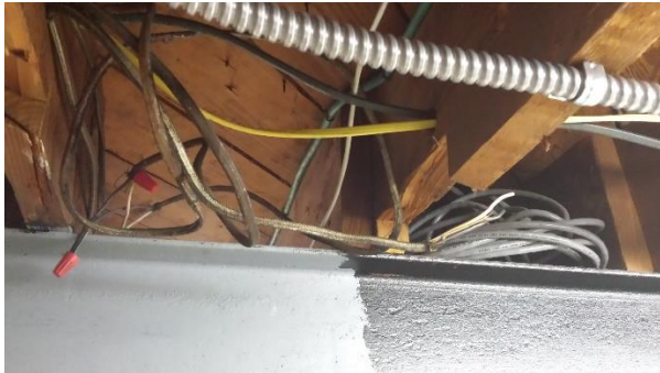
Old Administration Building (101T) – Outside Restroom 5
