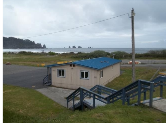
Culture Building (102T) – Picture Shows the NW Corner of the Building
