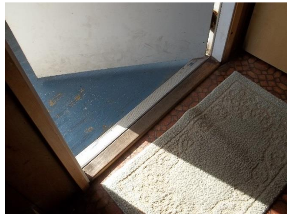
Culture Building (102T) – Exit Doorway from Classroom 1
