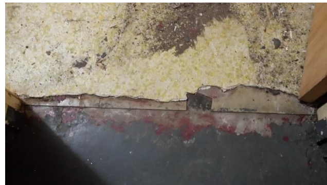
Old Administration Building (101T) – Restroom 5 Doorway Layer Detail
