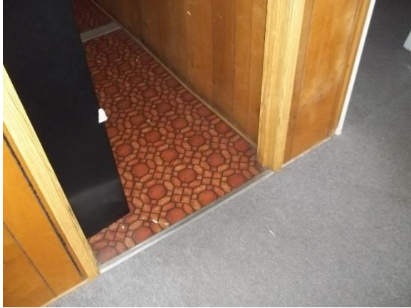
Culture Building (102T) – Hallway to Classroom 5
