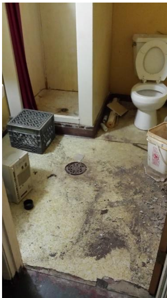
Old Administration Building (101T) – Old Basement Restroom 5
