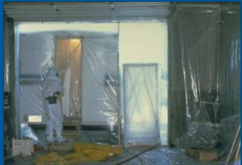
Asbestos abatement area contained and enclosed
