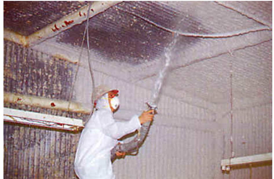
Structural Steel and Deck Coating
